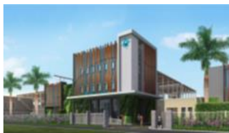
Coloane WTP 30,000m 3 /d
