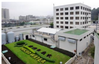
IV WTP 180,000m 3 /d
